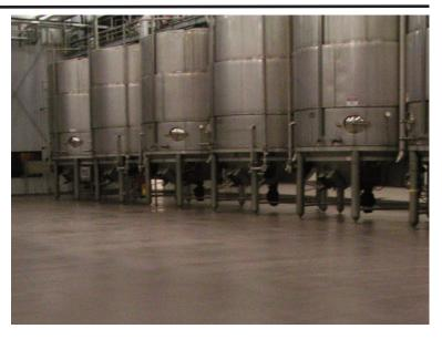
According to the people at Vincor Canada wine environments present numerous challenges. The floors must withstand spills of acids found in the wine making process as well as the caustics used to clean up those tough spills. Maintenance is important and there is no time to stop production for repairs and floor replacement. While the public thinks of wine as a slow process, production in this busy winery does not stop.
