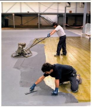
A power trowel is used in wide open areas to produce a smooth, flat surface. The floor is attractive, easy to maintain, and makes it easier to operate wheeled vehicles.
