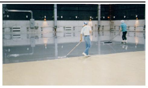
Part Two: A second primer layer follows the first to provide conductivity and an additional seal.
