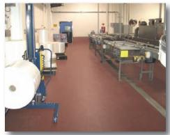
ing facility, with ex- Stonclad UT replaced an unsafe, failing epoxy brewing floor in Cold Springs Brewery's batching
